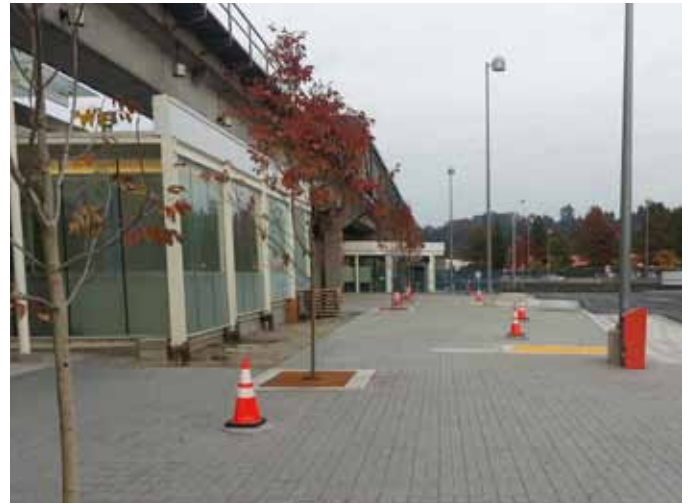
Construction phase, fall 2013
