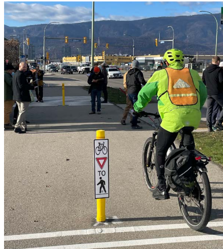
Figure 27: Example of Low-risk Channelization with Flexible Delineator Post, Kelowna, British Columbia
