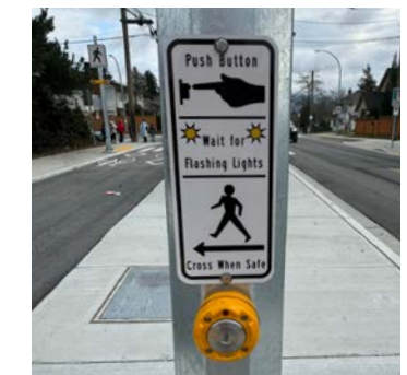
Figure 39: Example of Pushbutton at Actuated Flashing Beacon, Mission, British Columbia
