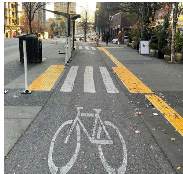
Figure 12: Detectable 'Bookend' at End of Island Platform Using Flexible Delineator Posts, Vancouver, British Columbia
