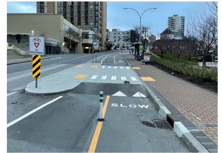
Figure 24: Bikeway Raised to Sidewalk Level Adjacent to Island Platform, Nanaimo, British Columbia
