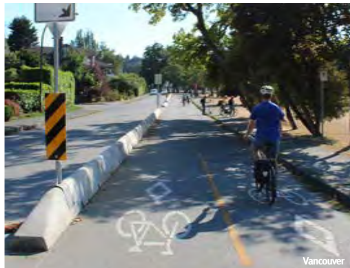
Figure 39 – Concrete barrier protected bicycle lanes
