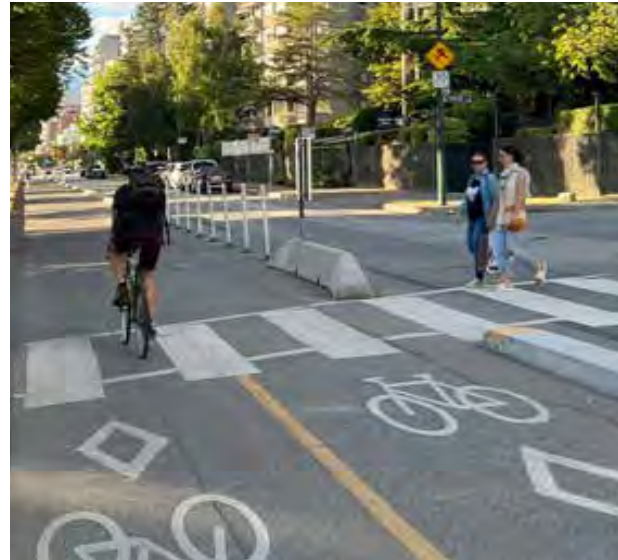
Figure 40 – Hybrid solution with extruded curbs, flexible delineator posts, and concrete barriers to provide a bi-directional protected bicycle lane (Beach Avenue, Vancouver)
