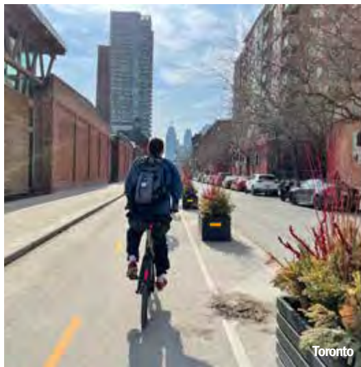
Figure 36 – Planter boxes used as standalone protection (left) or in conjunction with concrete curbs to provide additional protection
