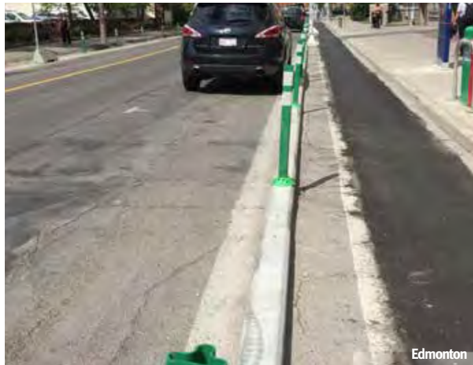
Figure 37 – Pre-cast curb protected bicycle lanes with flexible delineator posts atop the curbs
