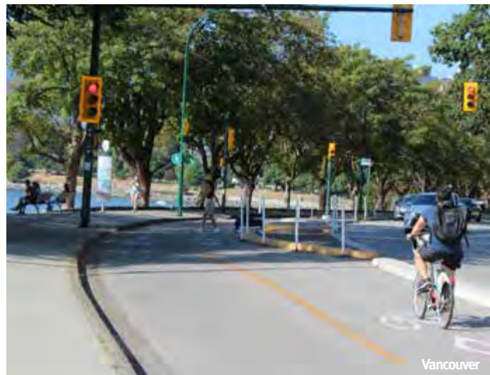
Figure 38 – Extruded curb protected bi-directional bicycle lanes
