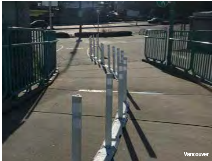
Figure 34 – Protected bicycle lanes with modular plastic curb protection
