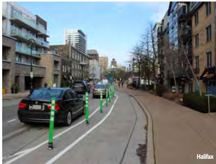
Figure 33 – Painted buffer protected bicycle lanes with flexible delineator posts
