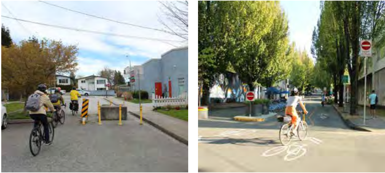
Figure 42 – Traffic diversion along neighbourhood bikeways in New Westminster (left) and Vancouver (right)
