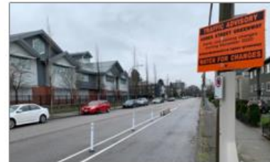
Agnes Greenway (interim solution) Location: New Westminster Length: 1.2 km Cost: about $100k + design fees Timing: Dec 2020; about 2-mos. to design, 2-days to implement Materials: road markings, flexible bollards, strategic concrete barriers, signage
