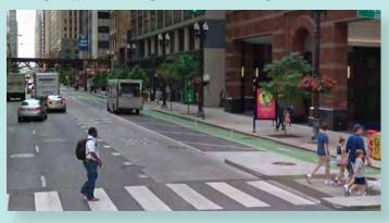
Figure C5.4: End of Transit Approach Lane with Separated Turning Traffic - Washington Street in Chicago<sup>2</sup>
