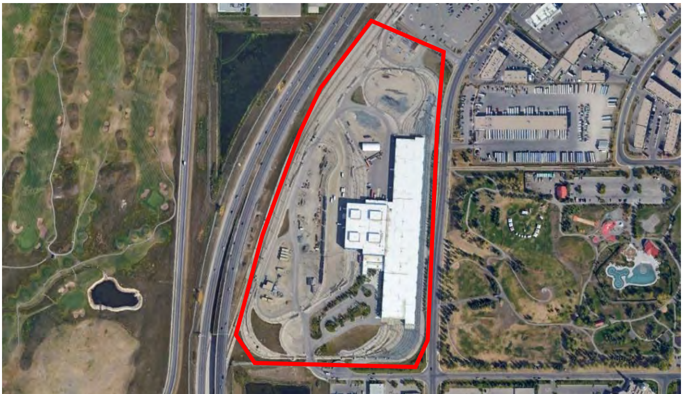
Figure 7-2: Oliver Bowen LRT Maintenance Facility, Calgary. Approximately 13 hectares with 2,800 linear metres of storage track. Stores 108 x 26m Siemens LRT vehicles. Site has abundant amounts of unused space.
