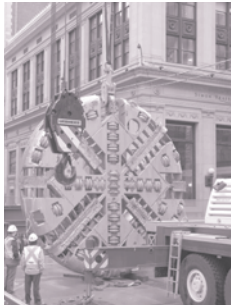
The tunnel boring machine, coming out of the ground last year.
