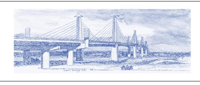
The bridge will be a low-profile adaptation of the Alex Fraser cable-stayed bridge. The Golden Ears Bridge has a simpler cabling system that will ease construction and maintenance, and its composite steel deck frame will be lighter and less expensive than more traditional concrete superstructure alternatives.
