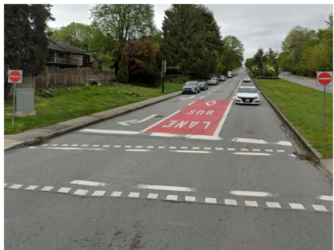
Offset transit lanes on West Keith Road maintain on-street parking near a commercial area.
