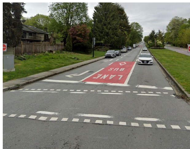
Offset transit lanes on West Keith Road maintain on-street parking near a commercial area.
