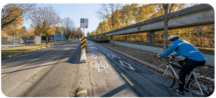
Simple protection with low concrete curbs offer protection to cyclists - photos by TransLink.
