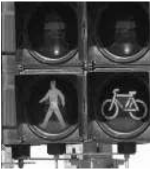
Perth bike crossing lights
