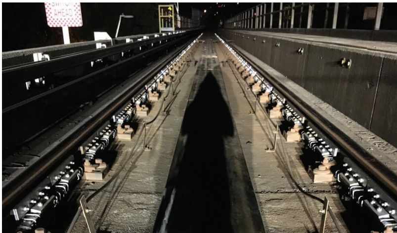
Figure 6 Nanaimo Outbound Track with Rail Dampers
