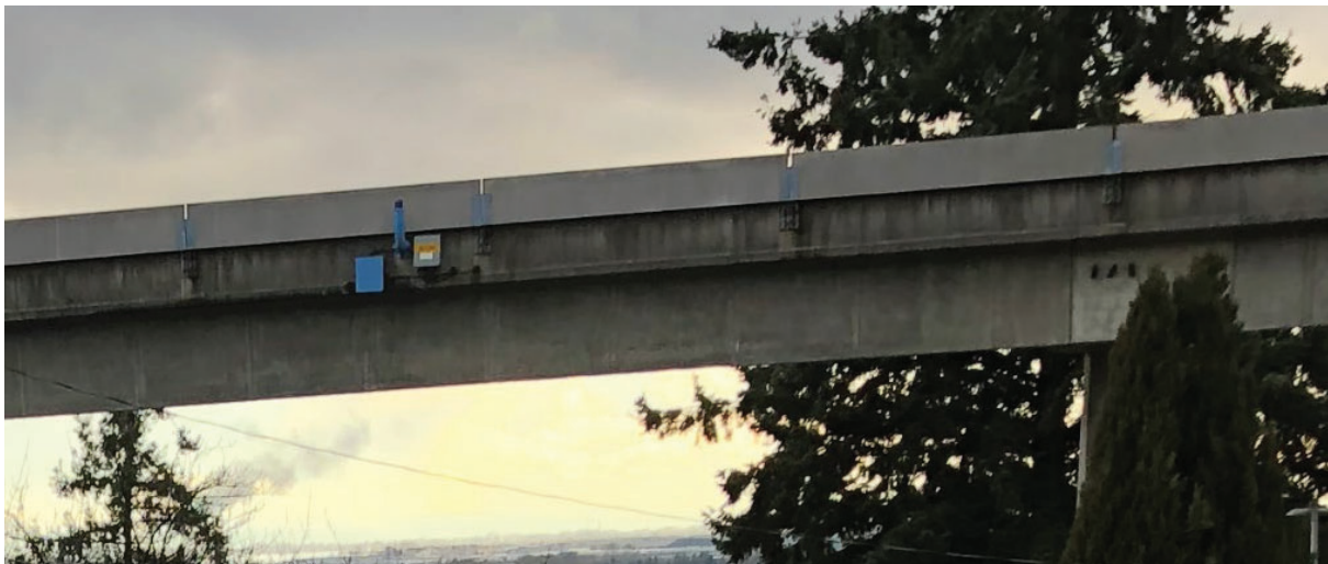
Figure 4 Example of SkyTrain Parapet Noise Barriers
