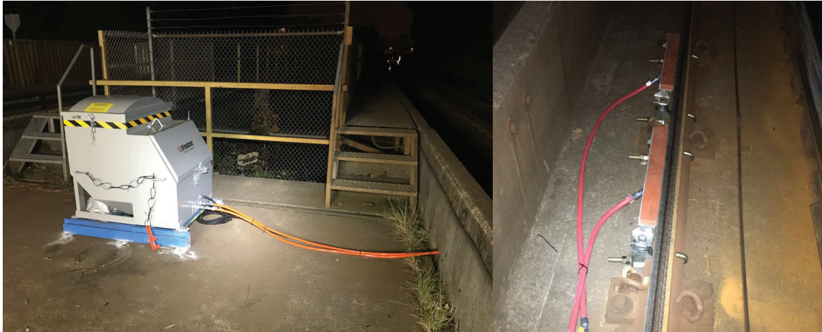
Figure 8 Pilot Study Wayside Applicator for Liquid TORFM
