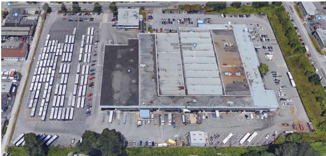
Figure 4 Burnaby South Transit Centre
